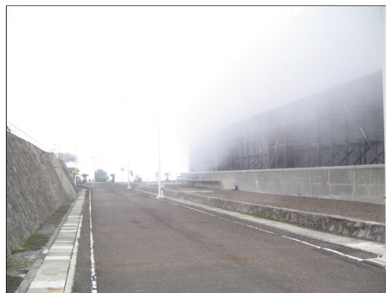
Figure 1: Major plume recirculation in Unit 1 CT.
