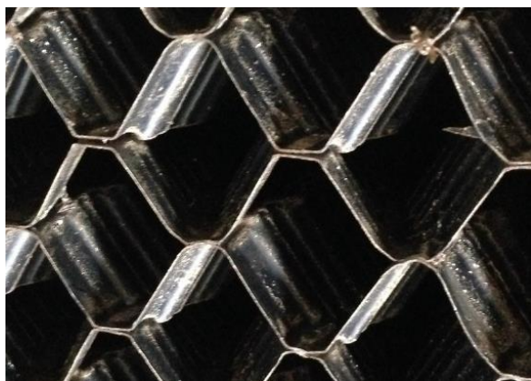
Figure 7: Unit 2 bottom of top layer of fill (Sep 2016)
