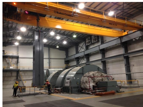
Figure 18: RHS column installation Unit 1.
