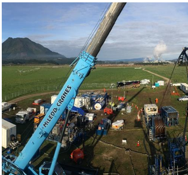
Figure 1: Layout of a well pad for chemical cleaning, note the large amount of equipment required for this clean utilizing a CTU.
