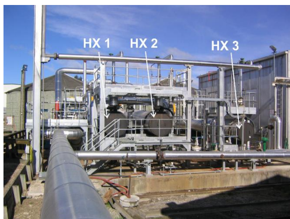
Figure 14: Tenon Two Phase Geothermal Heat Plant.
