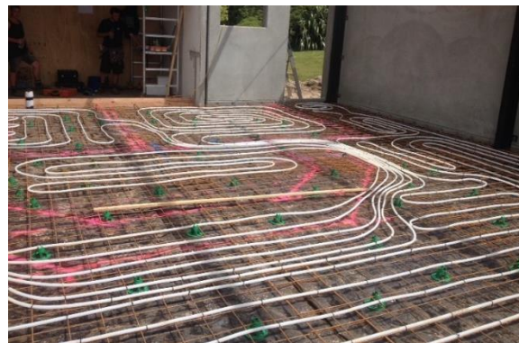
Figure 13 In slab hydronic piping at the Karapiti Kiosk (Photo courtesy Laser Plumbing Taupō)
