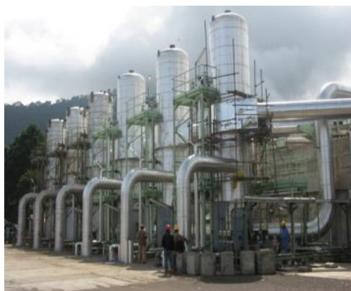
Figure 8: Two banks of three separators with integral water tanks for Wayang Windu units 1 and 2, each separator rated at 40 MWe. (Source: Purnanto and Purwakusumah, 2015)
