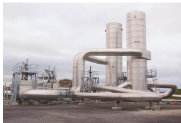
Figure 9: Flashplant 16 supplying Te Mihi Power Station on the Wairakei field, each separator is rated at 55 MWe (Source: Harwood, Koorey and Mann, 2015)
