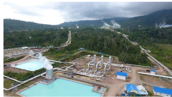
Figure 13: Overview of Unit 3&4 Central Separator station. Ulubelu 1&2 Power Station can be seen above the separator station while Ulubelu 3&4 Power Station can be seen to the right. (Source: PGE, 2017).
