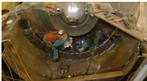
Figure 5: Replacing turning vanes in MPLP casing
