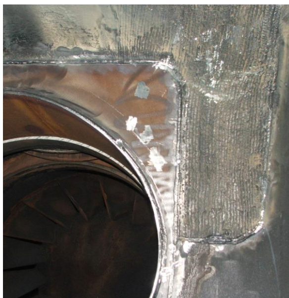
Figure 9: Full wall replacement and overlay weld repairs in LP manifold.
