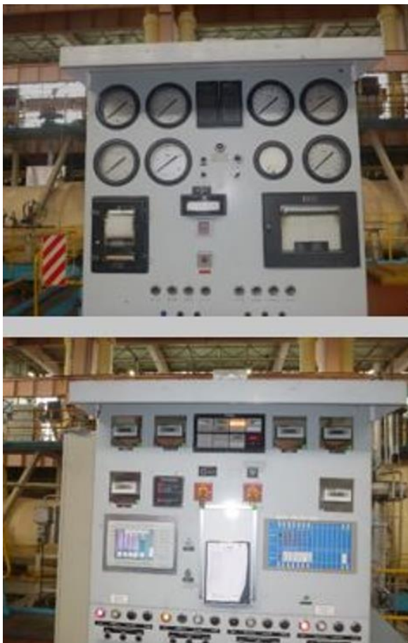
Figure 10: The original analogue TGB at top with current digital version below
