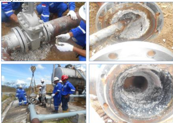
Figure 2. Major Scale inside the injection pipeline
