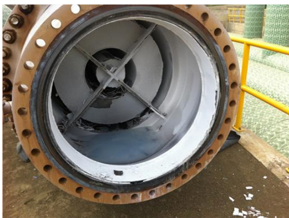
Figure 1: Scaling and brine carryover at Olkaria 1AU Pressure let down station silencer.
