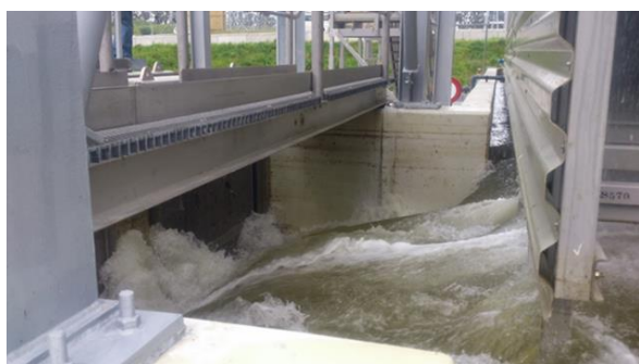
Figure 6: Initial hydraulic step at cold well inlet.
