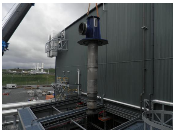
Figure 5: HWP withdrawal through removable roof.
