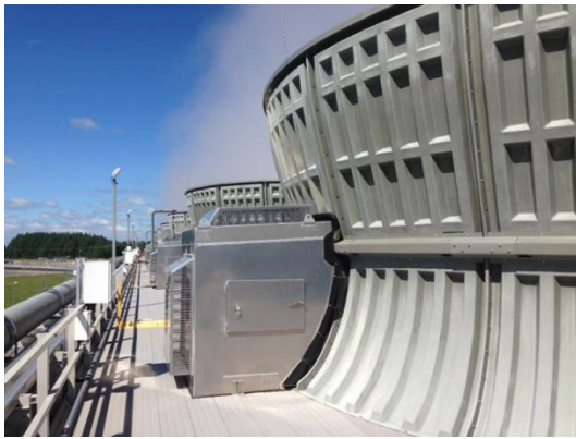
Figure 6: Permanent motor noise enclosures.
