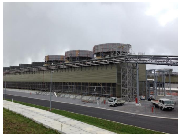
Figure 9: Temporary fan shroud to fans A, B & C.
