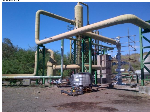
Figure 3: Well MT-36 and the combined Separator for brine flow from MT-36 / MT-43
