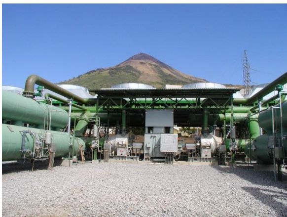
Figure 6: Ormat OEC bottoming unit, placed into service in October of 2002.
