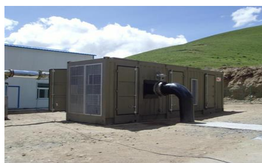
Figures 7 & 8: General Arrangement 500KW HSEPG unit, Yangyi Geothermal Project Stage 2, Tibet (grid connected 2012). Courtesy Demeter New Energy Ltd.
