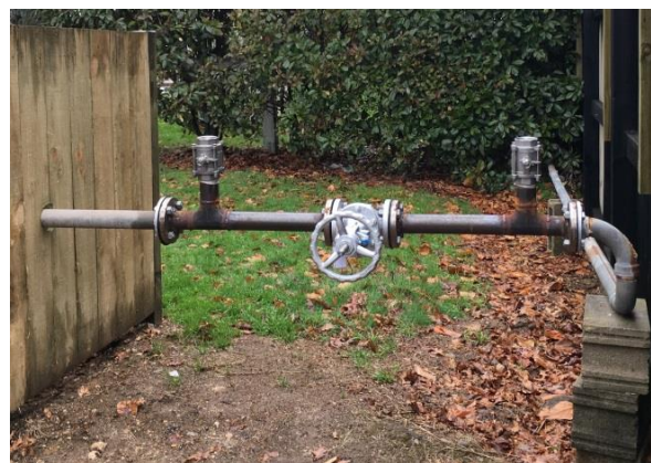
Figure 3: Flange-pipe permanent set-up at reinjection well.
