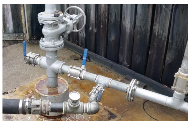
Figure 5: Connector to calorimeter near reinjection well.
