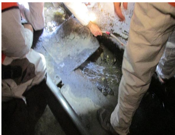
Figure 8: Seepage in the walls (left) and the floor (right) of the tunnel (from Kiwirail, 2013)
