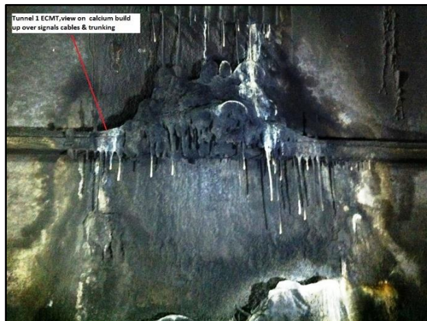
Figure 7: Travertine sinter that deposited near the wall seepage (from Kiwirail, 2013).
