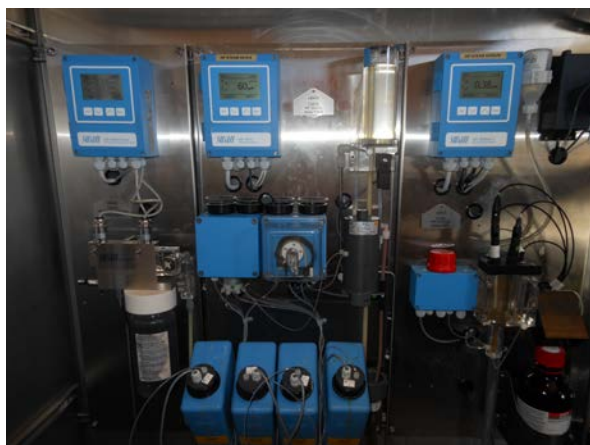
Figure 1: Steam Purity analysers at the Nga Awa Purua Geothermal Power Plant. Sodium, Silica, Conductivity and CACE shown.
