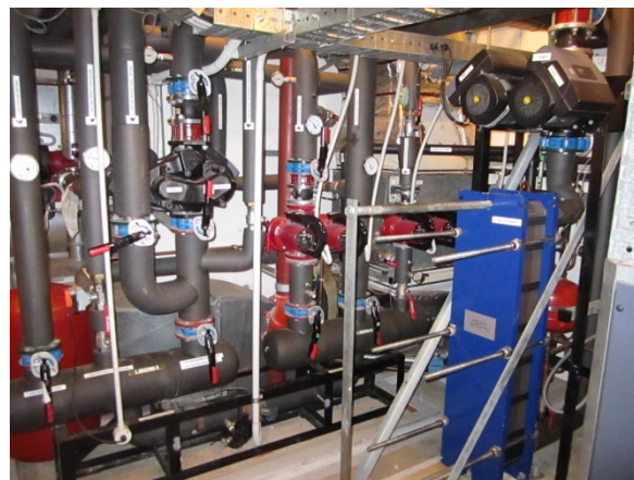
Figure 7: Partial view of plant room with the sea water heat exchanger in the foreground (some plates are temporarily missing).
