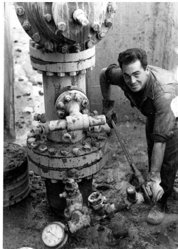
Figure 4: WK204 Wellhead equipment after removal of rig, 4.5.60
