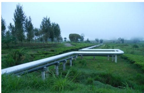
Figure 9 Installed HDPE line (black pipe) next to existing steel condensate line and insulated brine reinjection line
