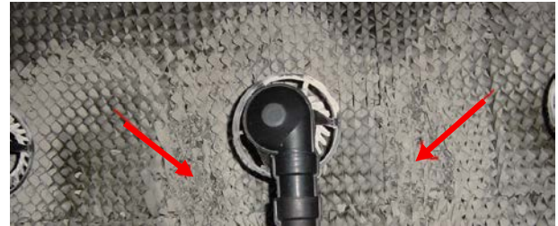
Figure 3. Areas of heavy sulfur fouling beneath spray nozzles result in uneven water distribution through the cooling tower fill, and damage to the fill (red arrows).
