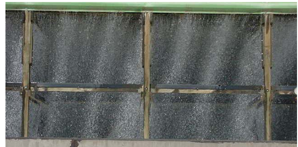
Figure 4. Channeled flow due to uneven water distribution beneath sulfur-fouled spray nozzles.
