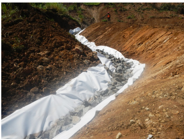
Figure 5: Temporary drainage from the upper pond
