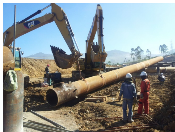
Figure 20: Lifting of pipe spool onto supports
