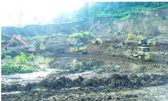
Figure 4: Clean-up of debris on the upper landslide area
