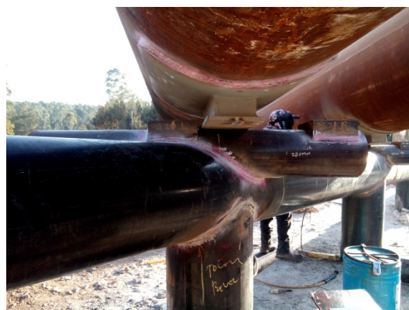
Figure 17: Special Bracket – Field Construction
