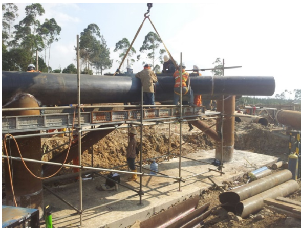
Figure 22: Construction of support frame LS-15
