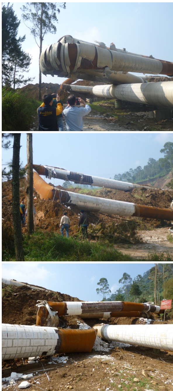
Figure 2: Pipelines Damaged by Landslide
