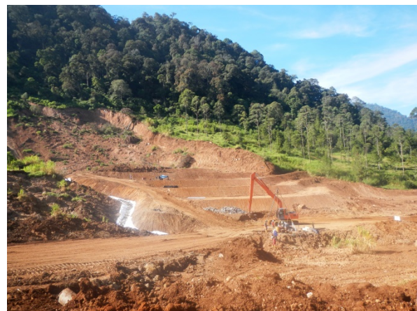
Figure 7: Reshaping to stabilize the upper part of debris
