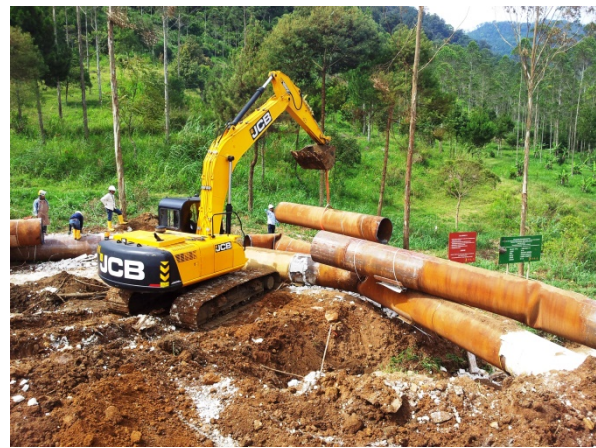
Figure 6: Damaged pipeline removal
