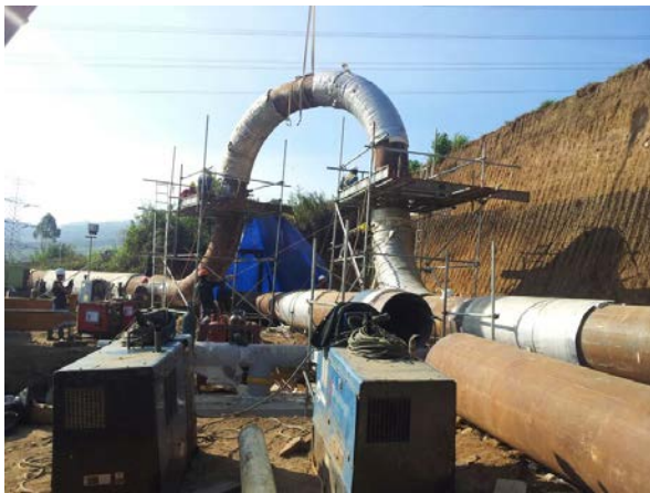
Figure 21: Fitting vertical loop (in Stage-1)
