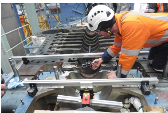
Figure 12: Measuring Diaphragm Bore Alignment
