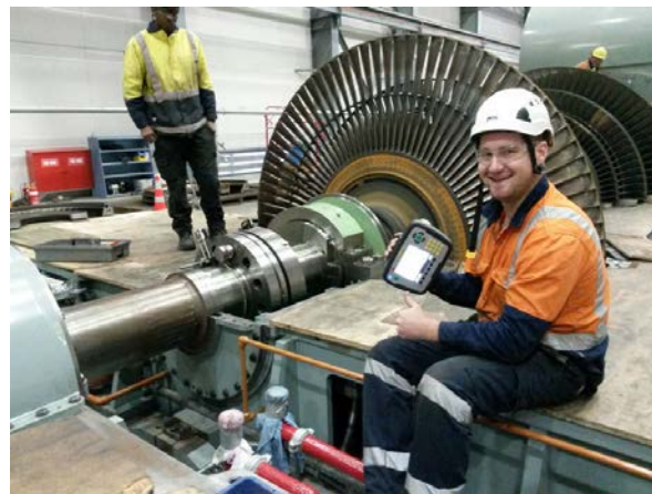
Figure 13: Measuring Shaft Alignment
