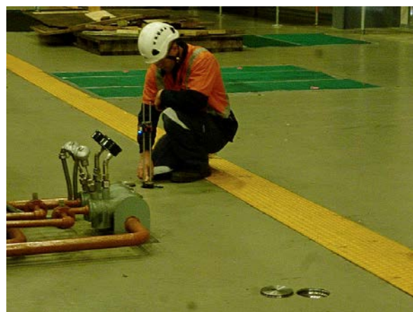
Figure 14: Measuring Embedded Plinth Datums
