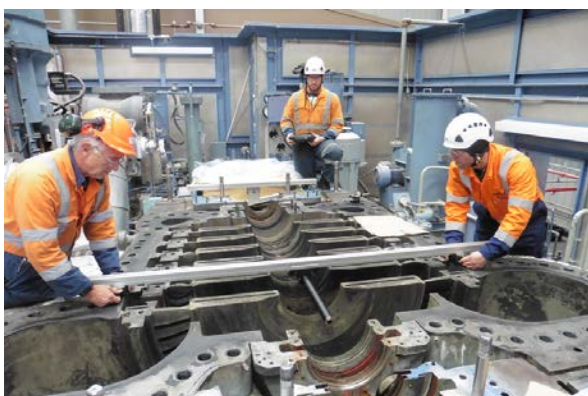
Figure 11: Measuring Diaphragm Bore Alignment
