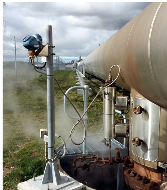
Figure 4: A guided wave radar device being used to monitor drain pot level. Note the insulation on the level bridge and the remotely mounted transmitter.
