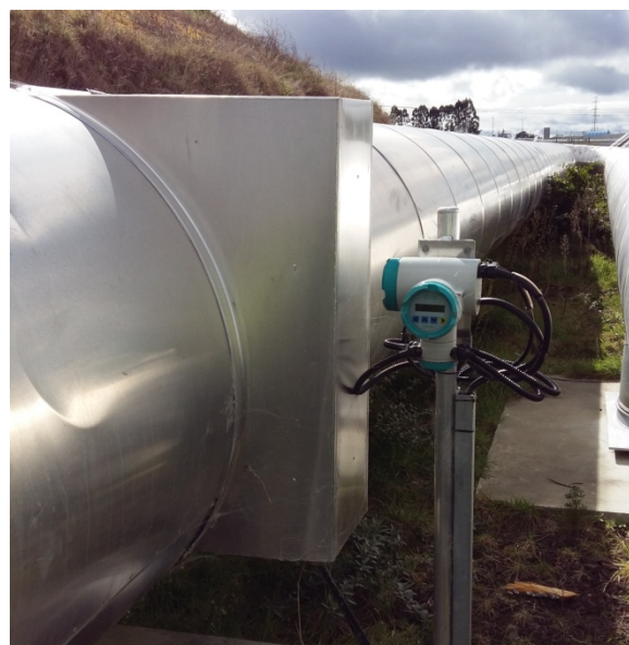
Figure 3: Ultrasonic flow meter with removable insulation and cladding covering the transducers.
