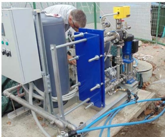
Figure 5 Above ground geothermal heat exchanger module
