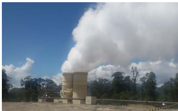
Figure 14: Well X-1 flowing at the separator after air compression
