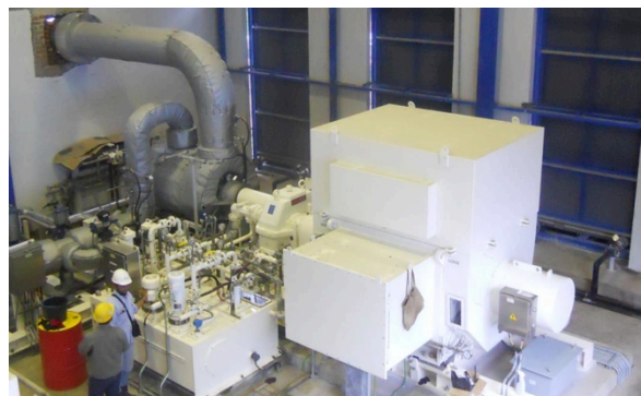
Figure 7: Unit 1 turbine generator set, inlet steam line and lube oil console during plant commissioning; auxiliary water coolers are installed in the background.
