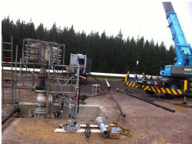
Figure 3: Perforation gun laid out ready to be run
