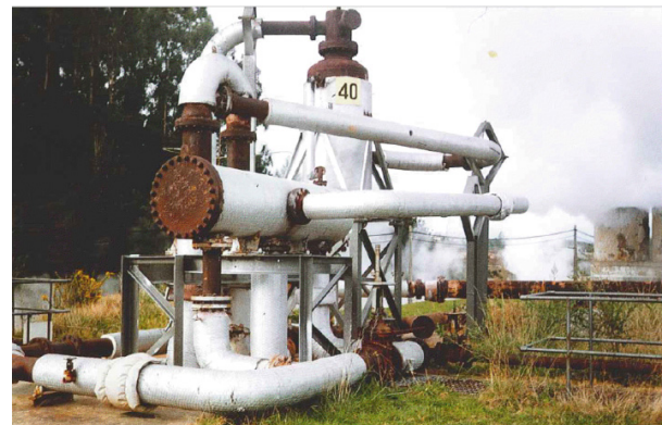
Figure 1: The U-bend Separator installed together with TOC Separator as seen in the Wairakei Field (Picture by Sadiq Zarrouk, 1997).
