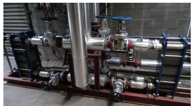
Figure 16: Primary heat exchange system in Taupo Hospital.
