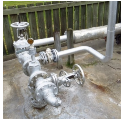
Figure 3: Self discharge well (RR 913).
