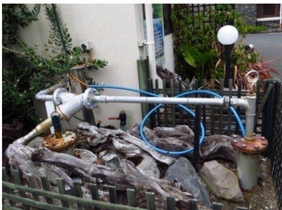
Figure 5: Down-hole pump well (RR 910 in the Wylie Court Motel).
