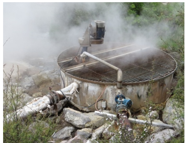
Figure 7: Concrete collection tank of hot spring water (S 952 in Holliday Inn, Rotorua).
