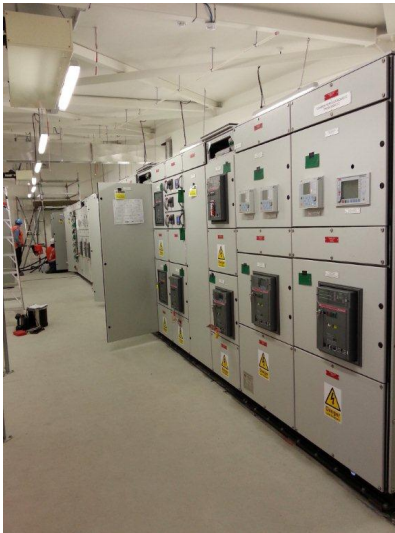
Figure 3c: Switchgear installation.
