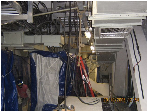
Figure 2: Example of congestion during erection activities in a typical electrical annex.
