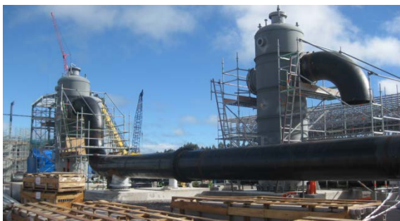
Figure 2.3.2: View of IP and LP Steam Scrubbers.
