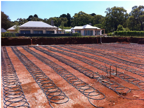
Figure 6: Part of the “slinky” system at Main Ridge
