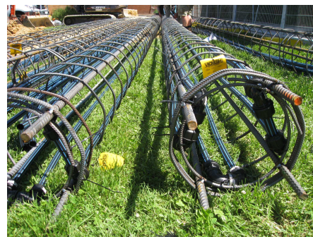
Figure 3: Pile reinforcing cages with ground loops ready for installation
