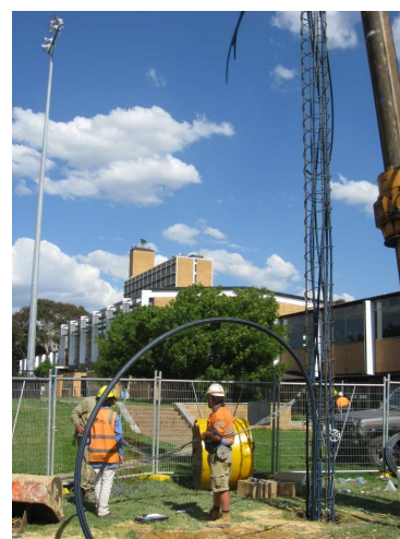
Figure 4: Installation of an energy pile at the Geothermal Test Facility
