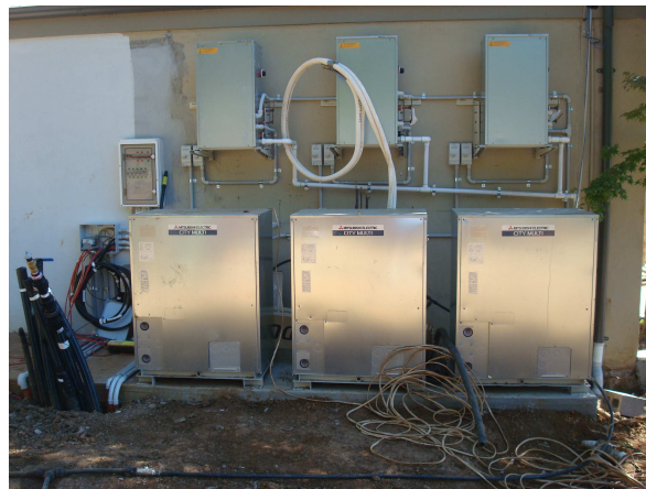
Figure 7: Mitsubishi GSHPs (note header pipes at left awaiting connection)
