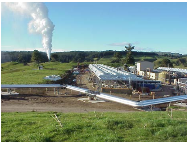
Figure 3 - Mechanical installation of machinery equipment and piping for Mokai geothermal power station at Mokai near Taupo in NZ undertaken by Fitzroy Engineering (Lovell, 2008)
