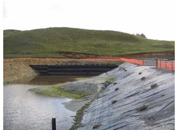
Photograph 1: Drained pond showing delta of cuttings
