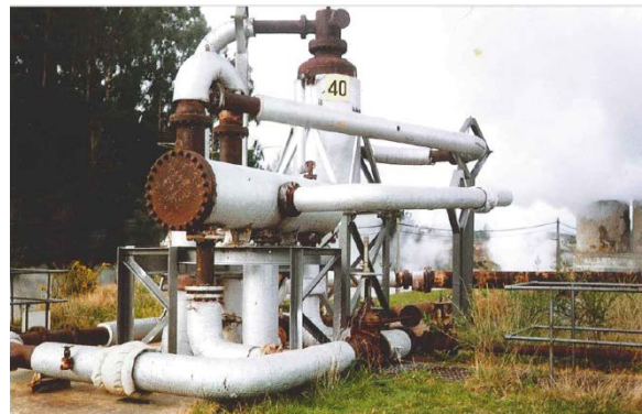
Figure 1: The U-bend Separator Installed Together with Top Outlet Cyclone Separator as seen in the Wairakei Field (Picture by Sadiq Zarrouk, 1997)
