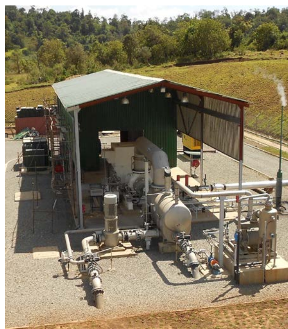
Figure 4. Eburru Wellhead Geothermal Power Plant in Operation
