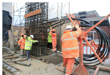
Figure 5: Ground loops in the reinforcing cage of a diaphragm wall during installation.
