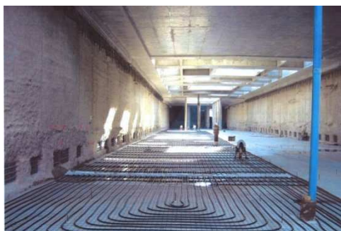
Figure 7: Horizontal ground loops in a mass concrete underground railway platform (Enercret, Vienna).
