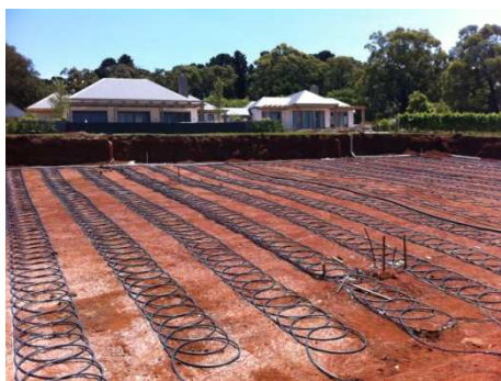
Figure 6: Large horizontal “slinky” ground loop installation before backfilling
