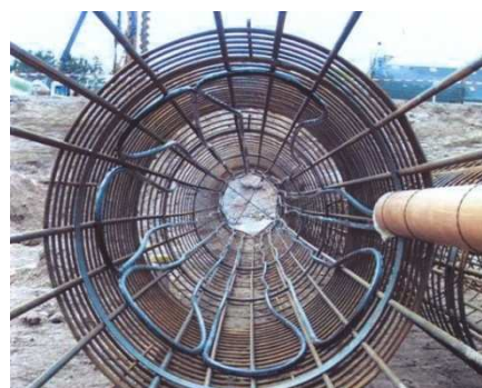
Figure 4: Ground loops in a reinforcing cage of a large diameter pile before installation (Enercret, Vienna).
