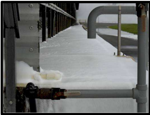
Figure 10: Foam inside the Kawerau cooling tower basin post unit trip
