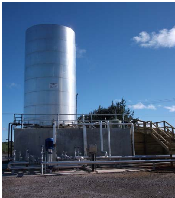
Figure 9: Feedwater tank and pump bank
