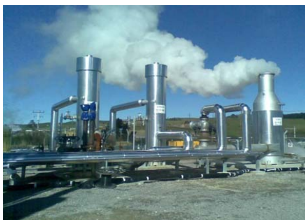
Figure 5: Cyclone separators and discharge silencer
