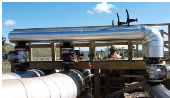
Figure 6: Separated geothermal water and condensed geothermal steam being returned via stab in's with diffuser cartridges to either 2 phase line for power generation (near side) or reinjection wells (far side)
