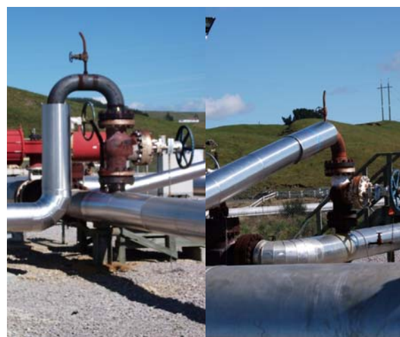
Figure 3: Top take off connections to Mk7A and Mk16 well head piping
