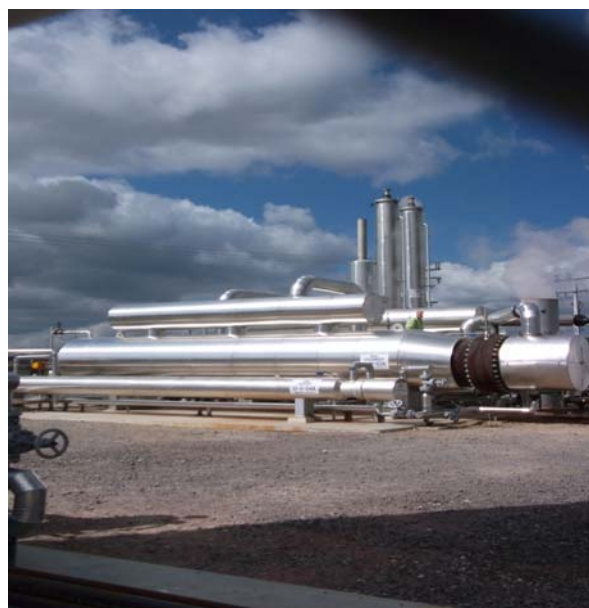
Figure 7: Heat Exchanger banks
