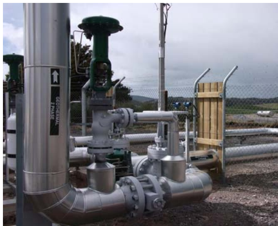
Figure 4: Split range pressure reduction valves supplying cyclone separators
