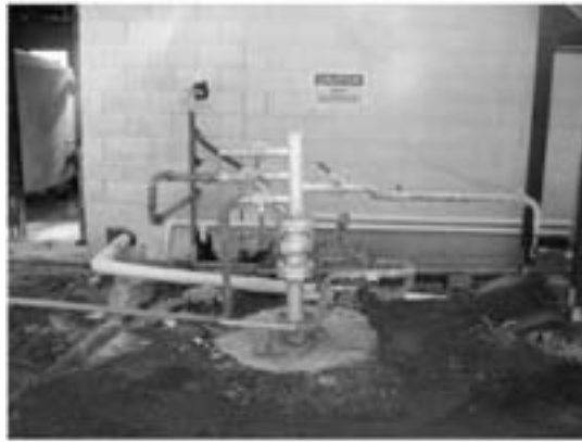
Figure 1. Well B8-N produces two phase (type-1) fluid (i.e. steam and liquid) to heat the public pools and 5 private pools.
