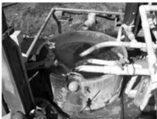
Figure 7. Steam condensates and fresh water mixing tank which provides mineral water to 5 private pools. Water leak can be observed.
