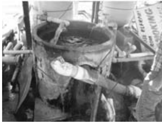
Figure 5. Type 2 water (from the Paurini pool) mixing tank with leakage indicated by arrows.
