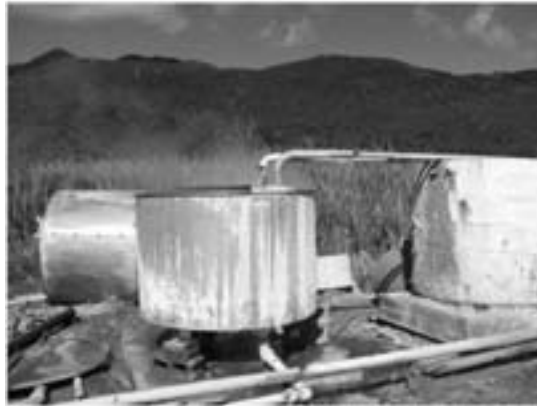
Figure 8. Current and former steam condensate tanks behind the bath-house. Also shown are the steel feeder pipe lines and the locations of corrosion due to the noncondensable gases (mainly H_2S ) in the bore water.
