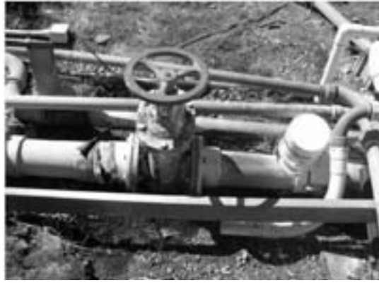
Figure 4. The PVC pipeline and 150 mm isolation valve for the Paurini pool water near the bath-house.
