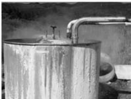
Figure 6. The condensate tank showing silica scaling, steam loss and over flowing of type 1 water.
