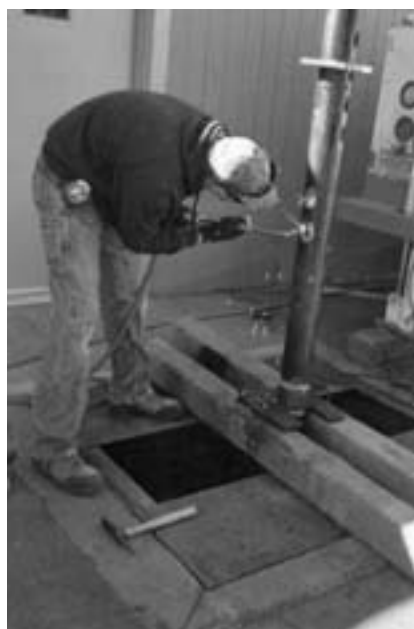
Figure 9: Cutting the 2.5-cm diameter perforations in the 10-cm diameter promoter pipe for the Klamath Medical Clinic
