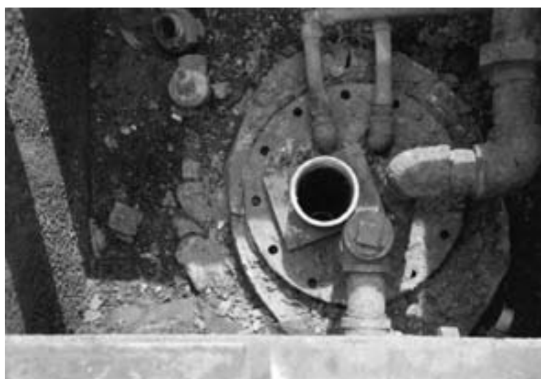
Figure 10: Looking down on the Klamath Medical Clinic well with the 6.4-cm diameter heating loop, the 2-cm diameter domestic hot water loop and the open promoter pipe suspended from steel plate
