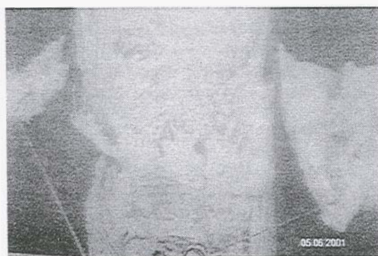
Figure 2. Fan-shaped silica deposits on the concrete divider between the two channels of the main drain. Field of view approx. 1.5 metre. Water flows from bottom to top of picture.
