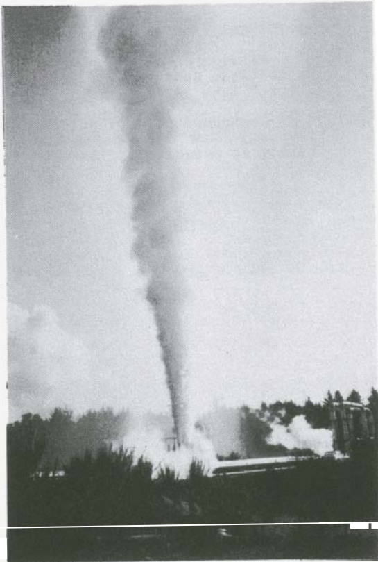
WEST STEAMFIELD SAFETY VALVES UNDER TEST
