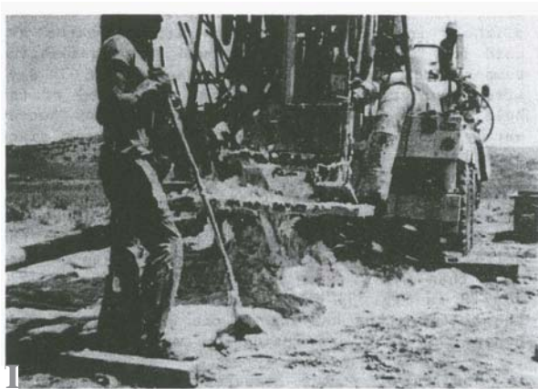
Fig. 2b: Aerated foam and cuttings (pumice) emerging from the top of the TG19 hole.
