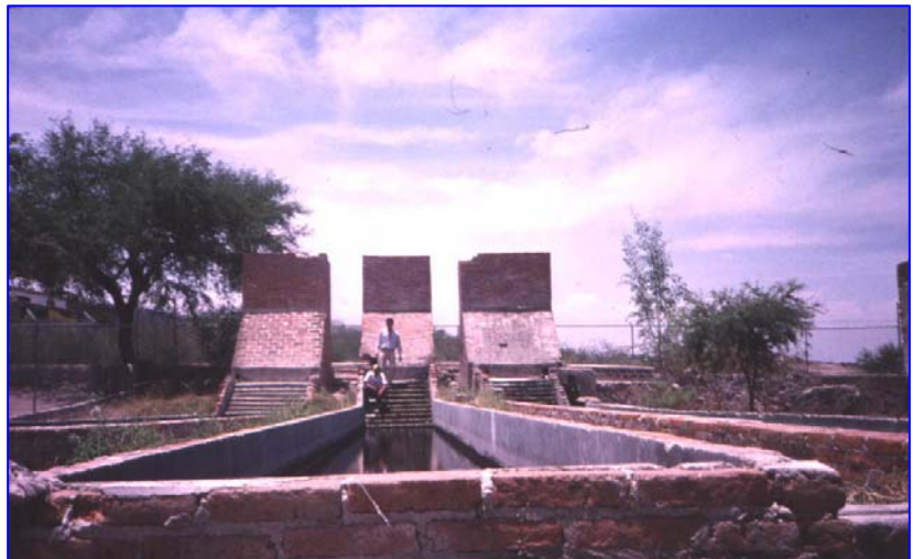
Fig. 6. The original water-collection troughs built at the spa. At the far end are the riffles the thermal waters tumbled over on leaving the aqueduct, the first of two cooling processes. Next the waters were mixed with cold water from a fourth trough until a good bathing temperature was reached.
