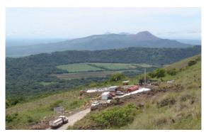
Figure 12: Slimhole drilling with a very small well pad enabled well CSS-01 at Casita to be drilled on very steep slopes. Water was carried by water tanker to the site.
