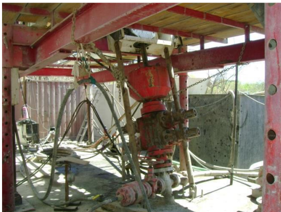
Figure 6: Blowout Preventer for slanted slimhole drilling
