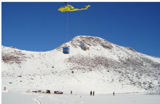
Figure 15: Helicopter supported slimhole drilling campaign at Laguna del Maule, Chile
