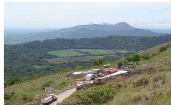
Figure 12: Slimhole drilling with a very small well pad enabled well CSS-01 at Casita to be drilled on very steep slopes. Water was carried by water tanker to the site.
