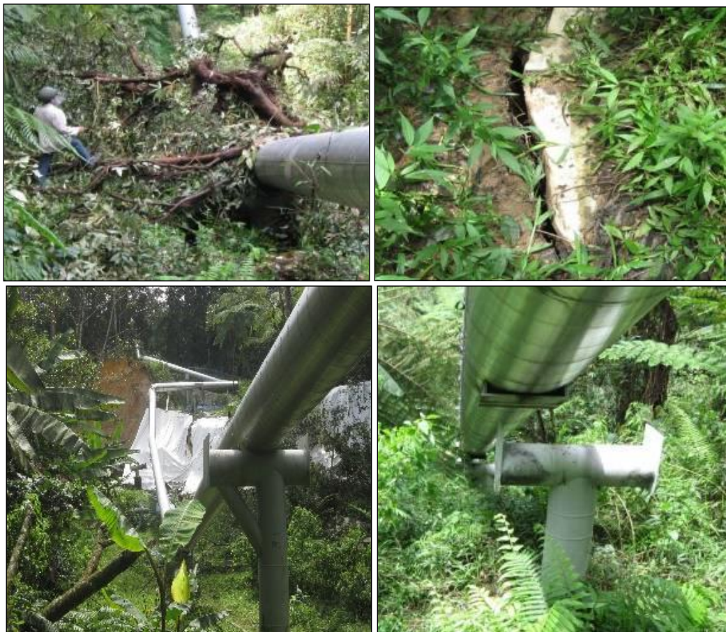
Figure 2. Fallen tree and pipe movement on Awi-14 brine line pipe
