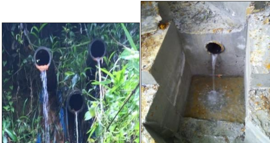
Figure 18. Completed installation of five (5) line of HDD at Awi-14 brine line pipe (left photo) and two (2) line of HDD at Awi-14 Well pad (right photo). Those HDD has successfully dropped ground water level
