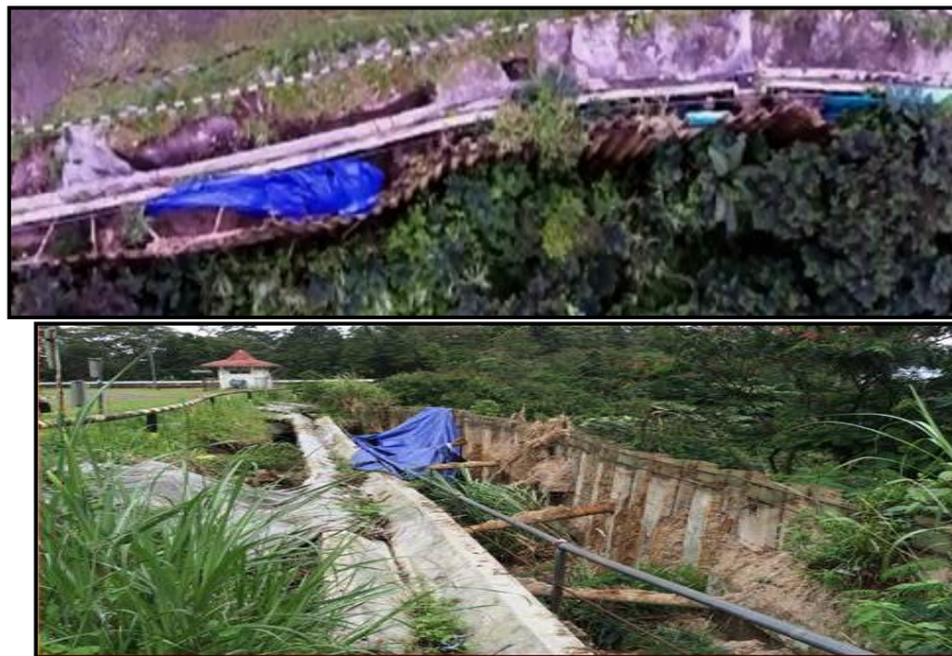
Figure 4. Soil subsidence and sheet pile shifting at Awi-14 well pad
