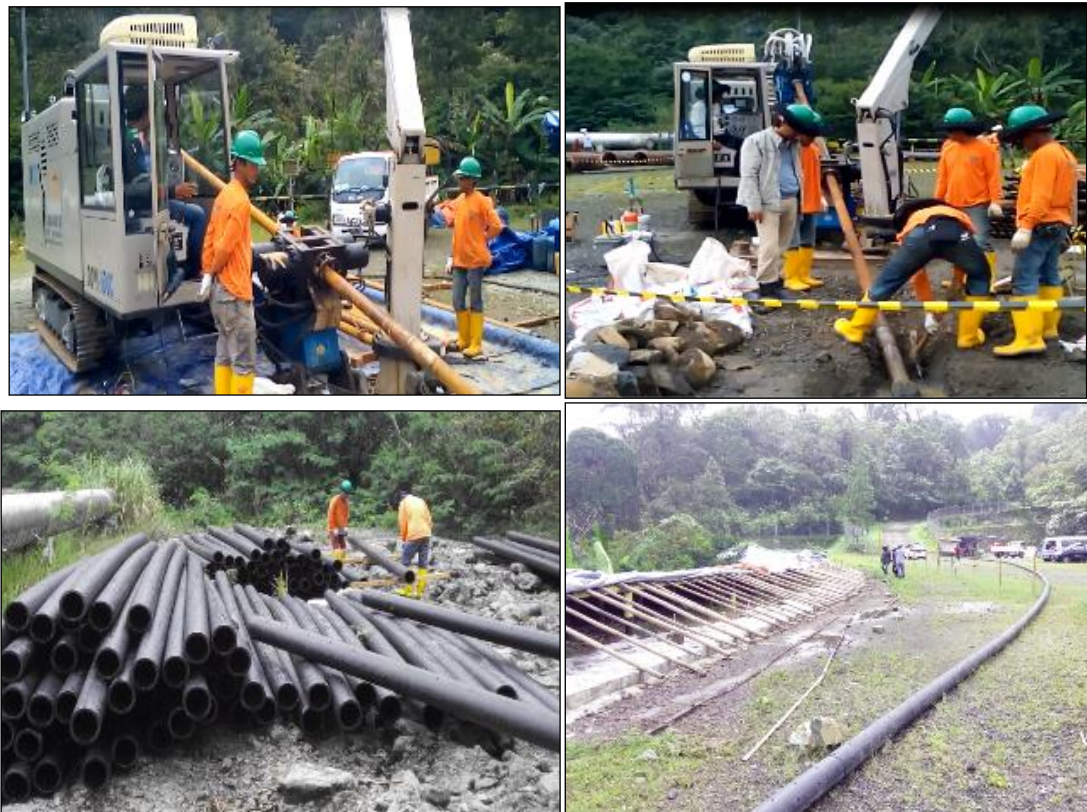
Figure 14. Horizontal drilling activity and HDPE perforated pipe 6" preparation before pulling back
