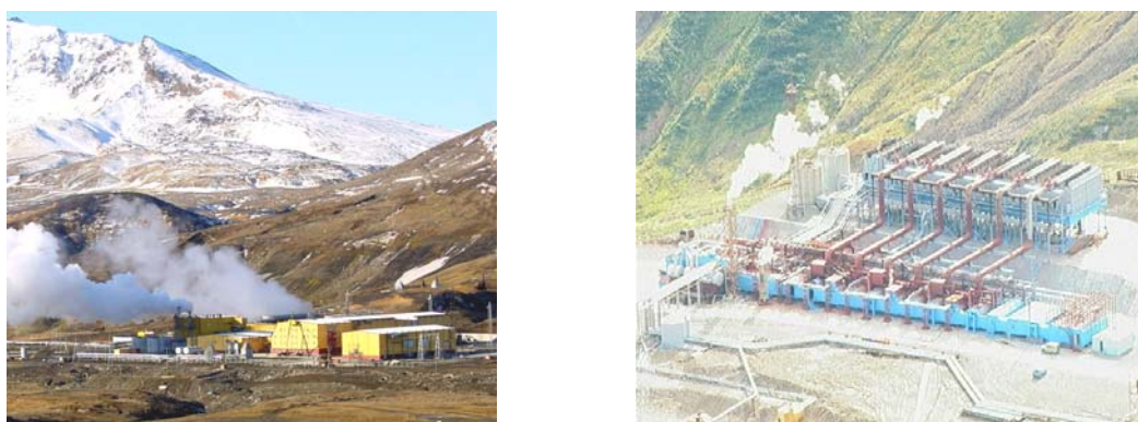
Figure 2: First environmental friendly 12 MW e (commissioned in 1999) Verchne-Mutnovsky GeoPP and the 1 st stage 50 MW e (commissioned in 2002) Mutnovsky GeoPP.
